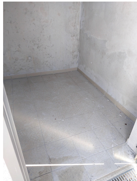
carrelage locaux techniques
